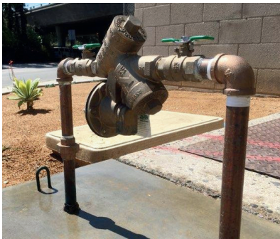
Reduced Pressure Principle (RP)
