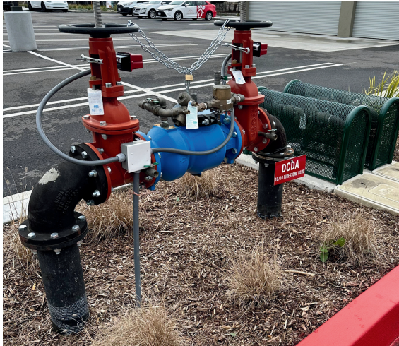
Double Check Detector Assembly
